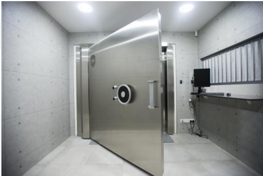
The 2.5 ton class I vault door to the silver depository
