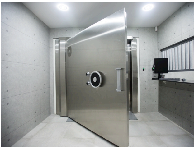
2.5 ton Class I vault door leading into the silver vault at The Safe House, Silver Bullion's subsidiary
